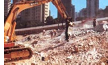
Reinforced Concrete Demolition & Concrete Cutting, Concrete Saws
